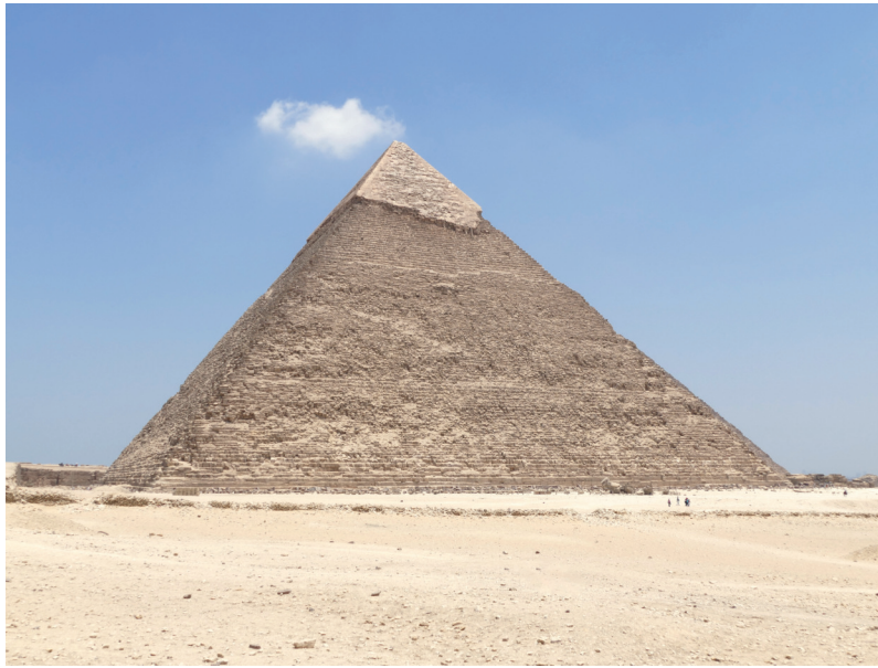
Fig. 11: The current state of the pyramid of Khafra shows that its casing had been dismantled from the bottom to the top.
