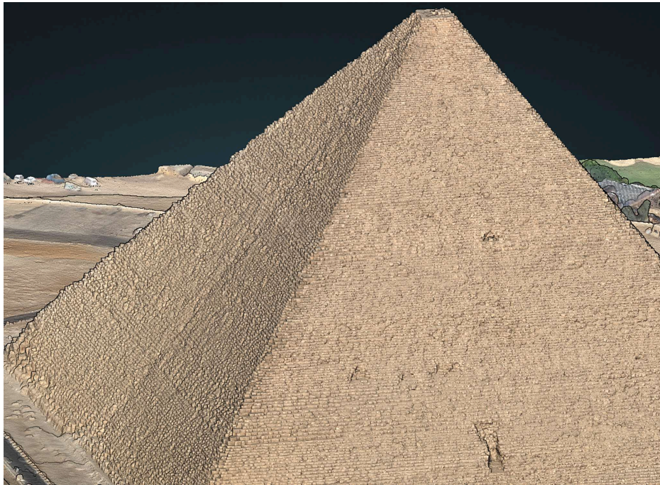
Fig. 9: Furrow following the apothem line of the western face of Khufu's pyramid (photogrammetry @ Label News, Iconem ).
