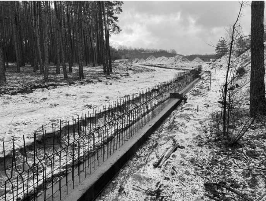
Figure 1: Documentation of current construction works at Sobibór, photo by Wojciech Mazurek.
