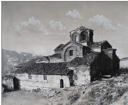
Fig. 2: Church of St. Clement, Ohrid, FYROM. View from the southeast, unknown photographer, undated (early 20 th century), collection of the Photographic Archive of the Department of Art History, University of Vienna. Digital image available at http://phaidra.univie.ac.at/o:526660 (accessed 19.5.2017), CC BY 4.0 license .
